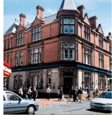
LLOYDS TSB BANK, 26-28 REGENT STREET, WREXHAM
